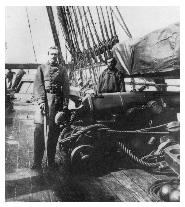
Figure 12 - Running rigging and breeching rope "Hawser-Laid", right-handed.
