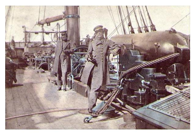
Figure 13 - Running rigging and breeching rope "Hawser-Laid", right-handed.
